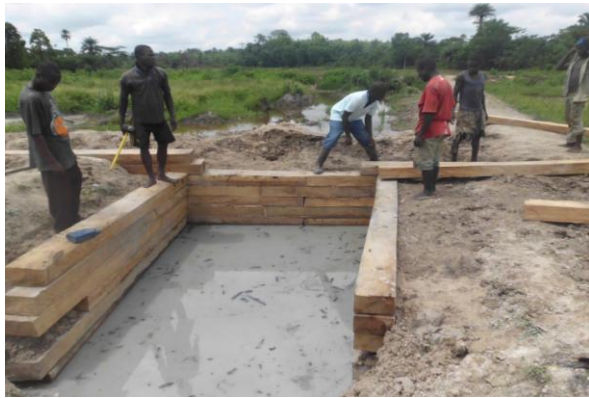
Update view of Zayglay spillway downstream
