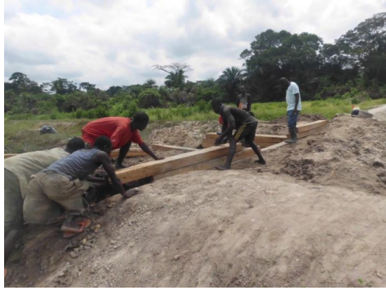
Construction of spillway
